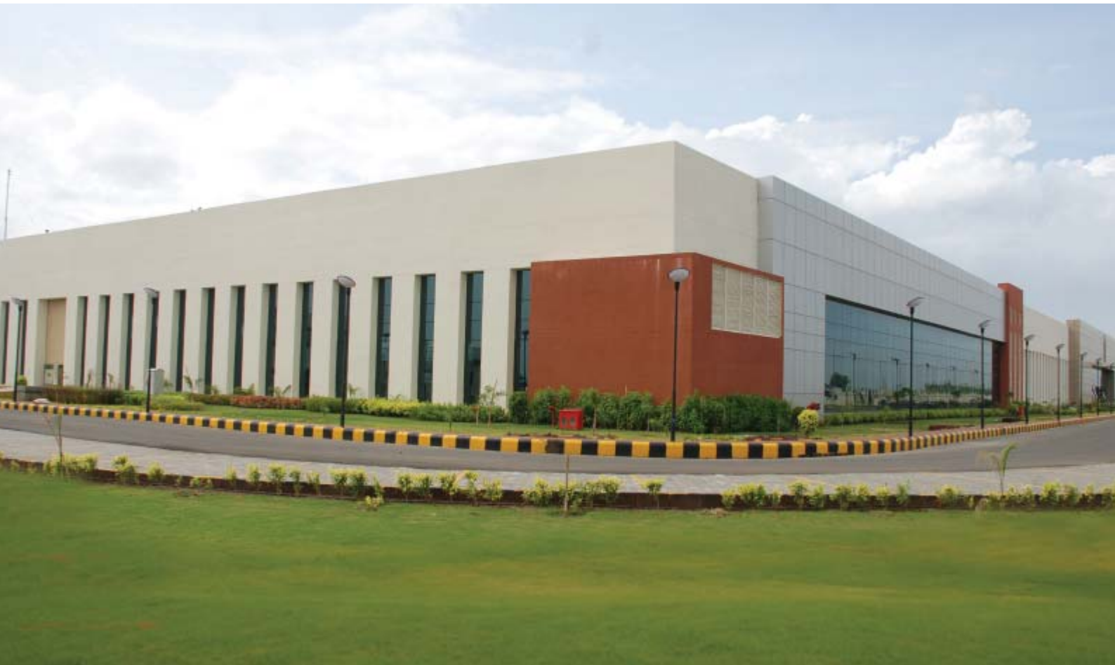
Switchgear Factory, Baroda
