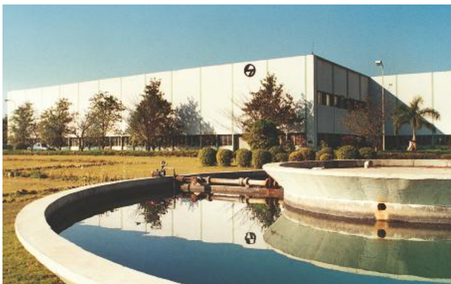
Switchgear Factory, Ahmednagar
