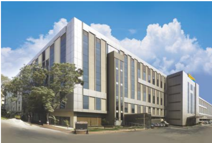
Switchgear Factory, Mumbai
